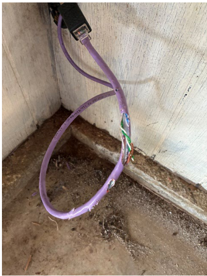
Wiring damage from ground squirrels inside offices and garage
